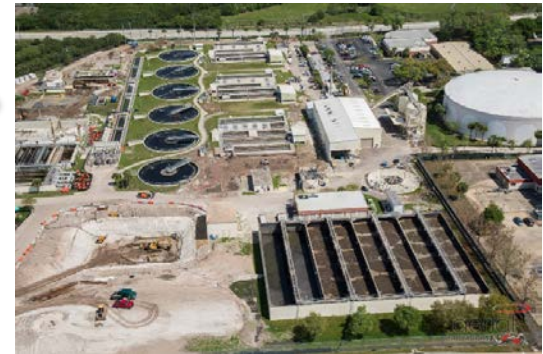
Transport to WWTF
