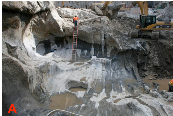
Figure 11 – World Trade Center site in lower Manhattan. A – 40' deep scoured plungepools. B – Filled with glacial till. C – Piece of wood dated at 49,500 BP. D – Found 2/3 of the way up, in a silt layer. E – Located within the dense till native to NJ, indicating flow from the NW.
