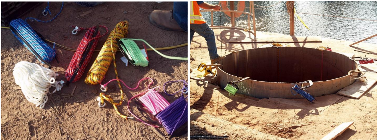
Figure 5 – Various ropes used with weights and C-clamps to hold ropes taught and vertical down the sides of the shaft in order to video each compass rose direction with depth calibration. Analysis of the color-coded videos allowed us to generate an accurate flat 2-D map of the interior of the rock socket.
